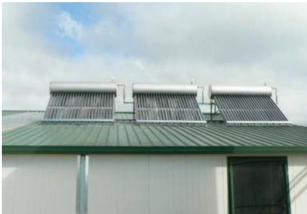
Figure 4.8 : Solar water heating installed at a farm dairy.
